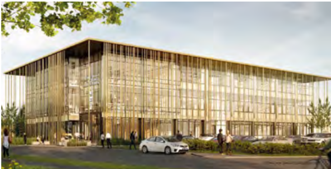
Food Science Facility Palmerston North
