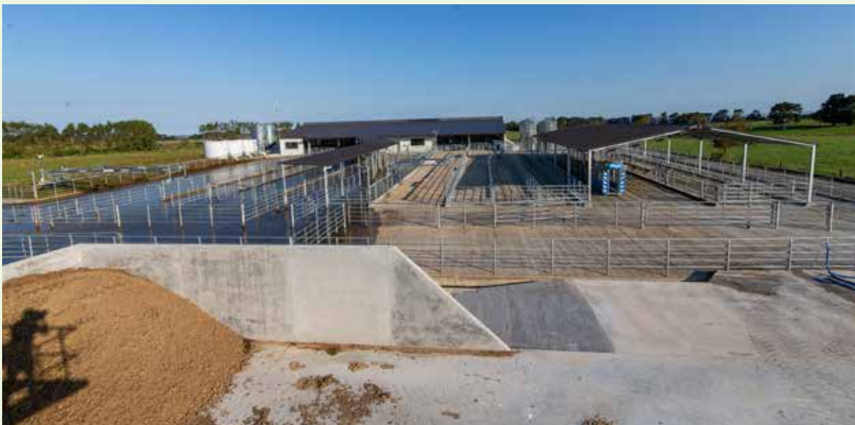
The Dairy 4 Farm development at Massey University in Palmerston North. Shown is the covered veterinary area (left), multi-lane feeding pad (right), and rotary milking operations (rear).
